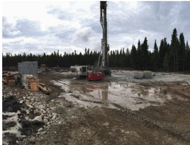
Piling to ensure the durability of the Women's Shelter in Waskaganish
