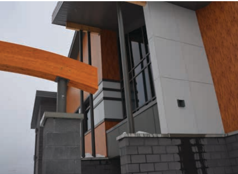
The Women's Shelter in Waswanipi is completed
