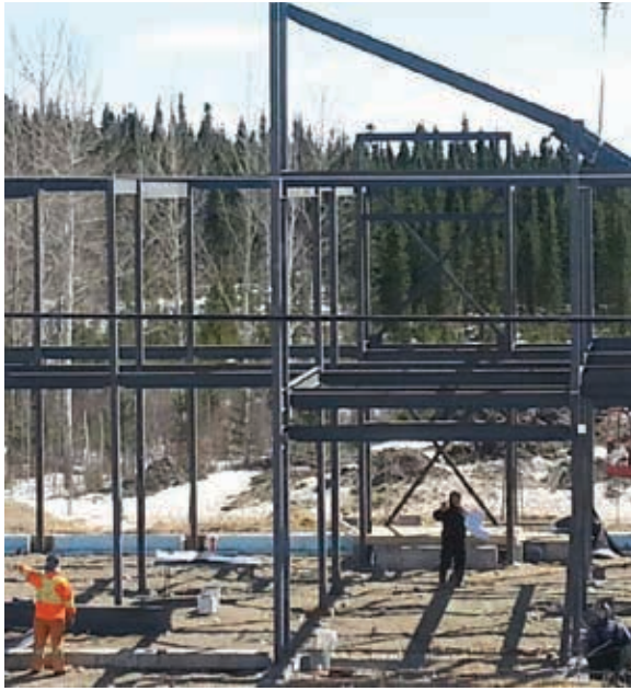
Building the Women Shelter in Waswanipi
